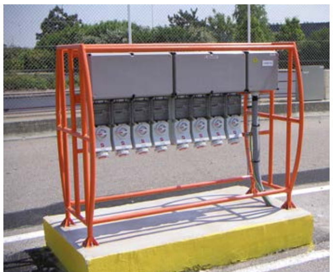
Container Terminal, Le Havre – France
