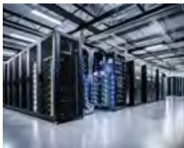
Power your Data Center
