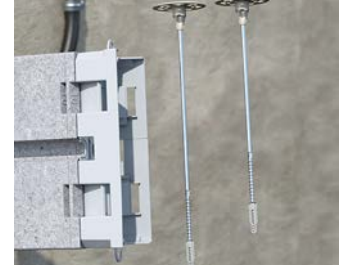
Remove the side lugs from the screw dowel. Note the different lengths!
