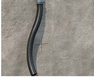
Masonry with conduit exit.
