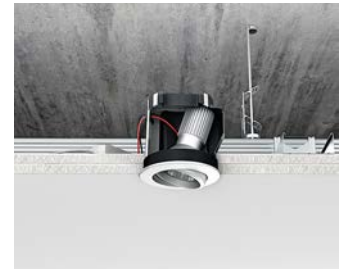
...and installing plasterboard.
