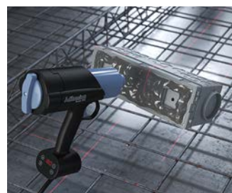
Fixing by means of hot glue.
