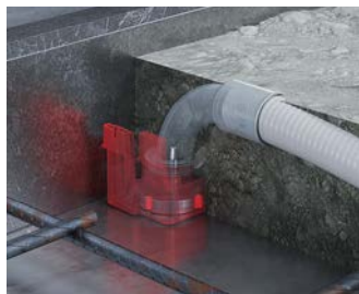
...the new wall-ceiling transitions 90°,...
