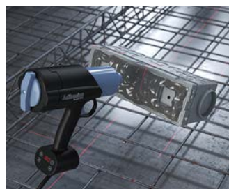
Fixing by means of hot glue.
